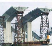
FOCUSING ON VALUE AND EFFICIENCY, SCHWAGER DAVIS, INC. DESIGNED AND SUPPLIED THE SUPERSTRUCTURE ERECTION SCHEME, HEAVY LIFTING EQUIPMENT AND AN ALL-NEW POST-TENSIONING SYSTEM FOR THIS MAJOR U.S. SEGMENTAL BRIDGE PROJECT. THE SKYWAY WAS SUCCESSFULLY COMPLETED IN DECEMBER OF 2006 AND THE PROJECT CURRENTLY RANKS AS THE LARGEST SINGLE POST-TESIONING CONTRACT IN U.S. CONSTRUCTION HISTORY.
