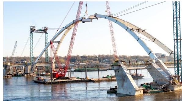
To facilitate temporary stay installation, SDI engineers specially designed threaded anchor ring nuts, post blocking devices, cable clamps, and performed proof load testing. The SDI shop then made necessary adjustments to the installation equipment (modifications, calibrations, setup) to suit the specially designed hardware.
