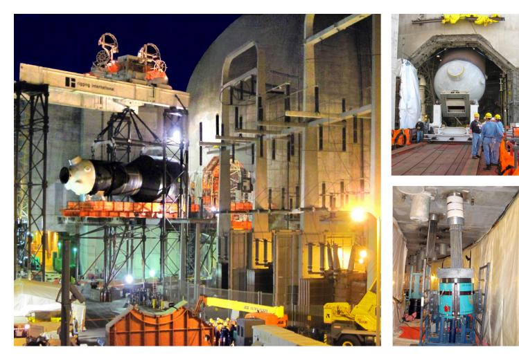
SCHWAGER DAVIS, INC. PROVIDES BECHTEL POWER CORPORATION WITH PROJECT-CRITICAL PT SOLUITIONS THAT MADE POSSIBLE A UNIQUE GENERATOR REPLACEMENT PLAN TO EXTEND THE POWERPLANT'S SERVICE LIFE. REMOVAL AND REPLACEMENT OF THE FIRST TWO OF FOUR 640-TON GENERATORS HAS BEEN ACHIEVED BY CUTTING A 28 FT. DIAMETER OCTAGONAL OPENING THROUGH THE HEAVILY POST-TENSIONED CONCRETE WALL OF THE UNIT 2 CONTAINMENT. THE SGR OUTAGE FOR UNIT 3 IS SCHEDULED TO COMMENCE IN SEPTEMBER 2010.
