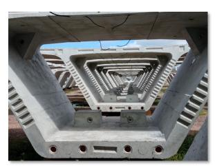
SDI's duct is visible here, and soon these precast segments will be lifted and tensioned together with post-tensioning strand (also supplied by SDI).
