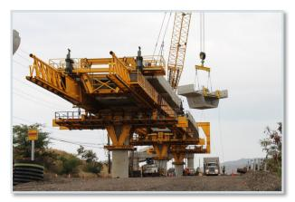
Precast segment of the elevated guideway being lifted into place. Post-tensioning will then be applied.
