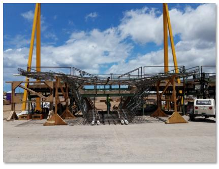
Note SDI's Corrugated PT Duct (white) running both longitudinally and horizontally in this form for a precast segment of the train's elevated guideway.
